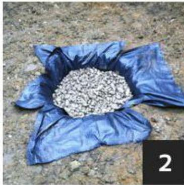
Line the hole with a permeable weed membrane (available at most DIY stores) and fill with scalplings, shingle or just crushed hardcore. The membrane will stop the hole silting up and allow water to collect and drain properly.
