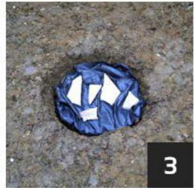
Finally wrap the membrane over the top of the hardcore/shingle/scalplings and lay some slabs on top to seal the top. You now have a very effective soak-away.
