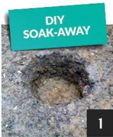
Dig a new hole at the bottom of the main hole about 2ft (60cms) in diameter and about 2ft (60cms) in depth.
